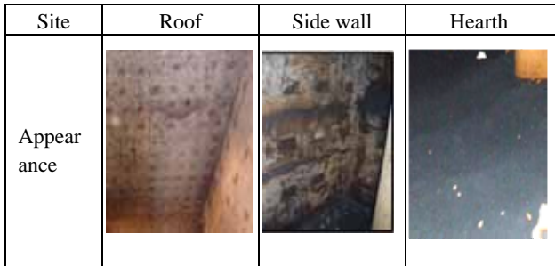
Figure 3 Photographs showing heating furnace refractories used for more than 30 years
