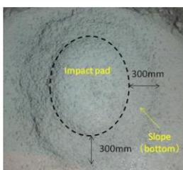
Figure 14. View of the third design combination for the impact pad and bottom refractory
