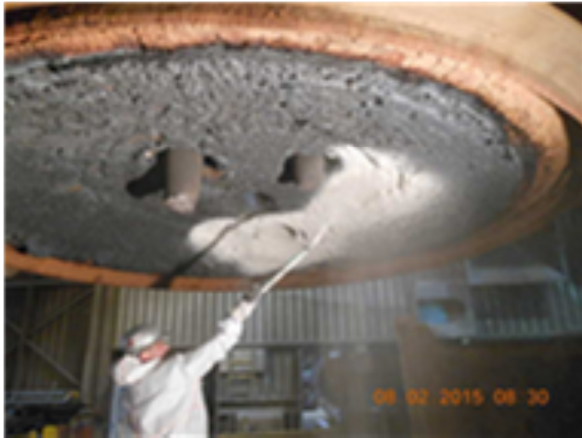
Fig.10: Repair of the EAF cover with the B-product
