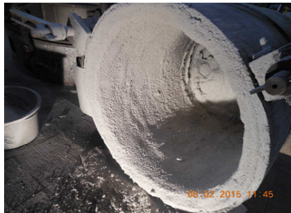
Fig.9: Ladle repair with the G- product
