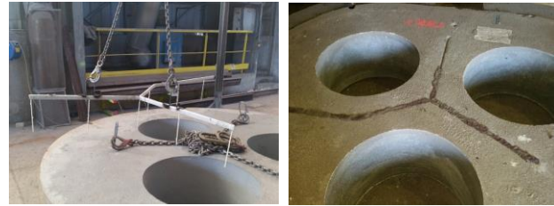
Fig. 3: Thermocouples introduction in delta roof.
